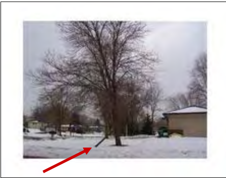
Would you consider this a reliable treatment to prevent this large ash from tipping any further? No? Good! Remove the tree. (Mike Meisch, UMN Extension )
