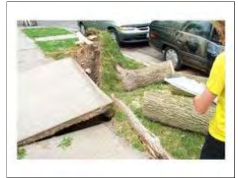
When large trees are left on narrow boulevards after street widening projects remove much of their roots, this is a pretty common scene for several years. (Gary Johnson, UMN Extension )
