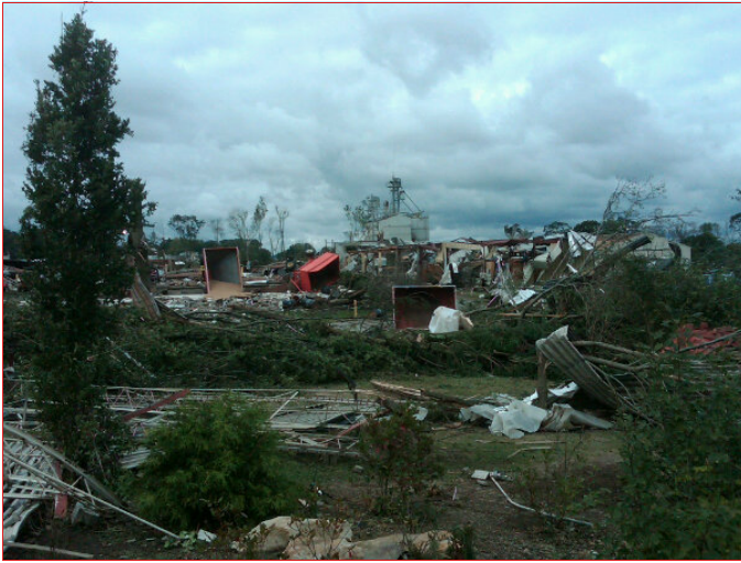
September 16, 2010 tornado damage
